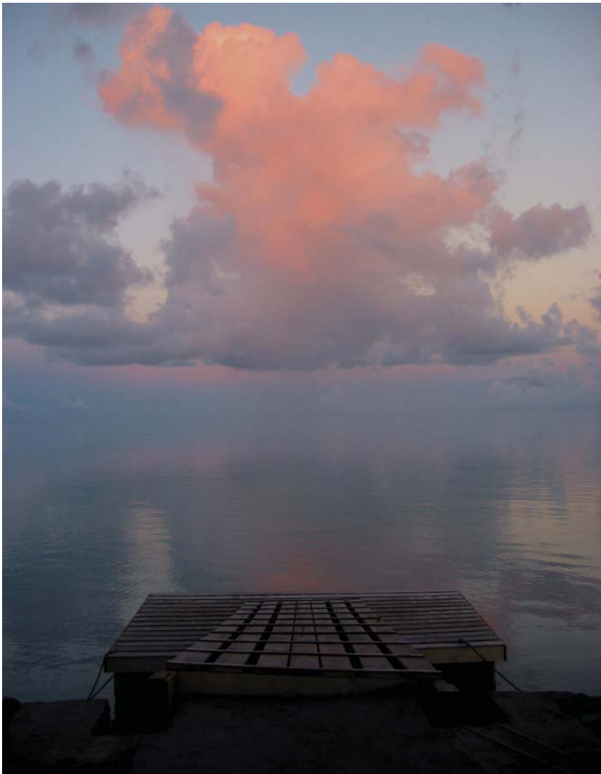
Photo 9: Coastal infrastructure vulnerable to sea level rise.
